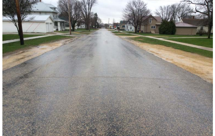
WILLIAMS STREET - SEGMENT 032 - HMA STREET - PCI=85
