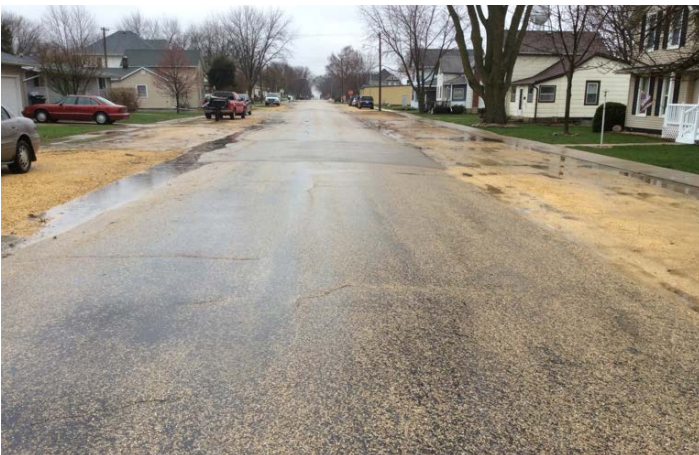
FULTON STREET - SEGMENT 041 - HMA STREET - PCI=44
