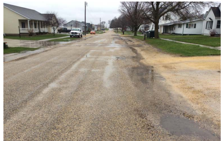
SUNNYSIDE STREET - SEGMENT 053 - HMA STREET - PCI=35
