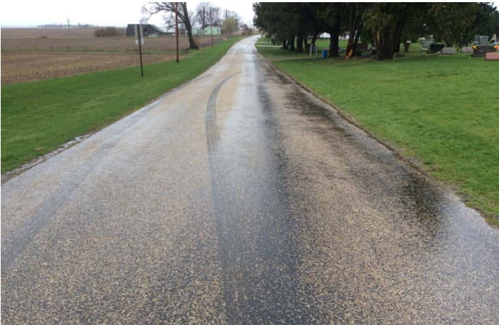
SUNNYSIDE STREET - SEGMENT 057 - HMA STREET - PCI=71
