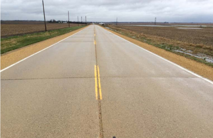
EAST STREET - SEGMENT 060 - CONCRETE STREET - PCI=85
