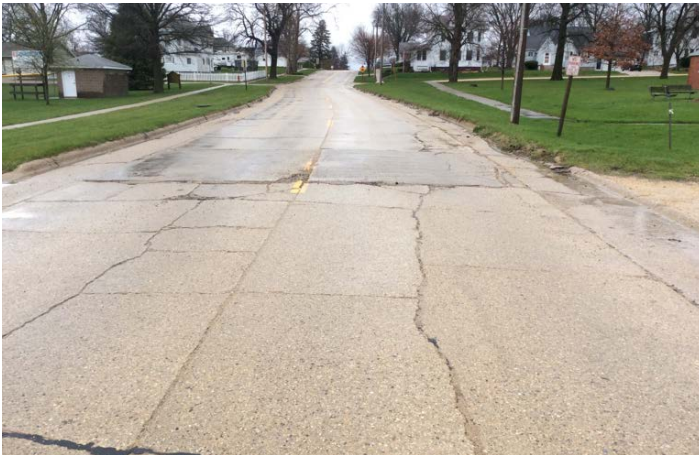
EAST STREET - SEGMENT 059 - CONCRETE STREET - PCI=43
