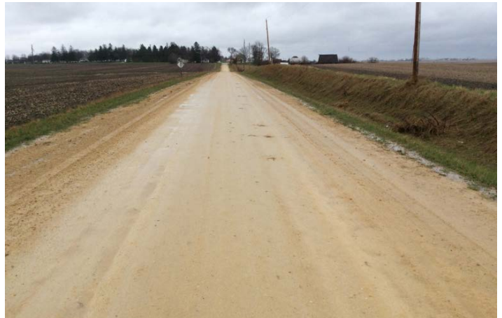
SUNNYSIDE STREET - SEGMENT 062 - GRAVEL STREET - PCI=50
