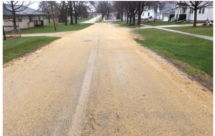
SUNNYSIDE STREET - SEGMENT 051 - HMA STREET - PCI=65
